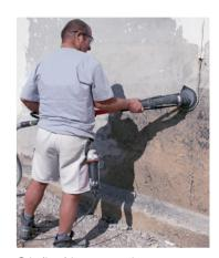
Grinding bitumen coating with PCD grinding disc
